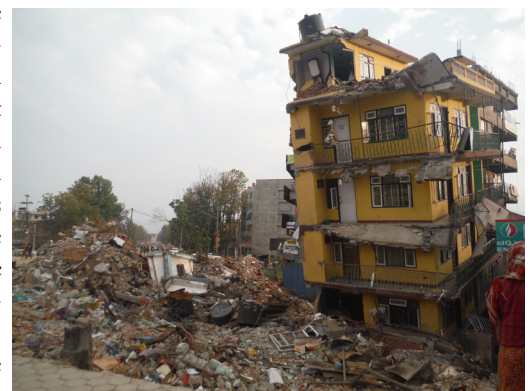
Unreinforced Brick Walls with Cast-in-place Concrete Diaphragm in Balaju, Kathmandu.
